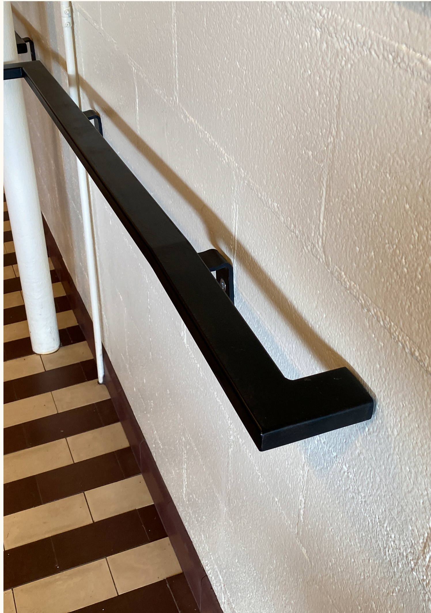
Close-up of railing end turning into wall
