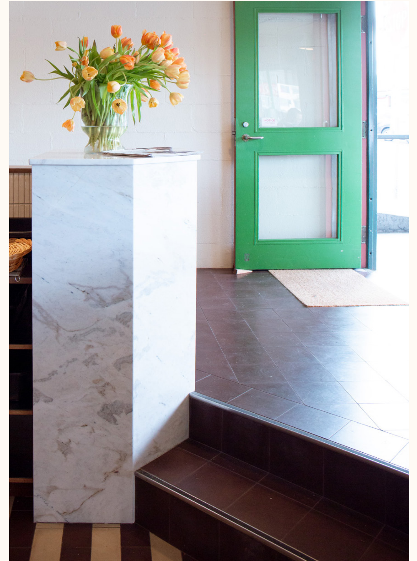
After: Stair schluter with non-slip grip. Coir mats remain the same
