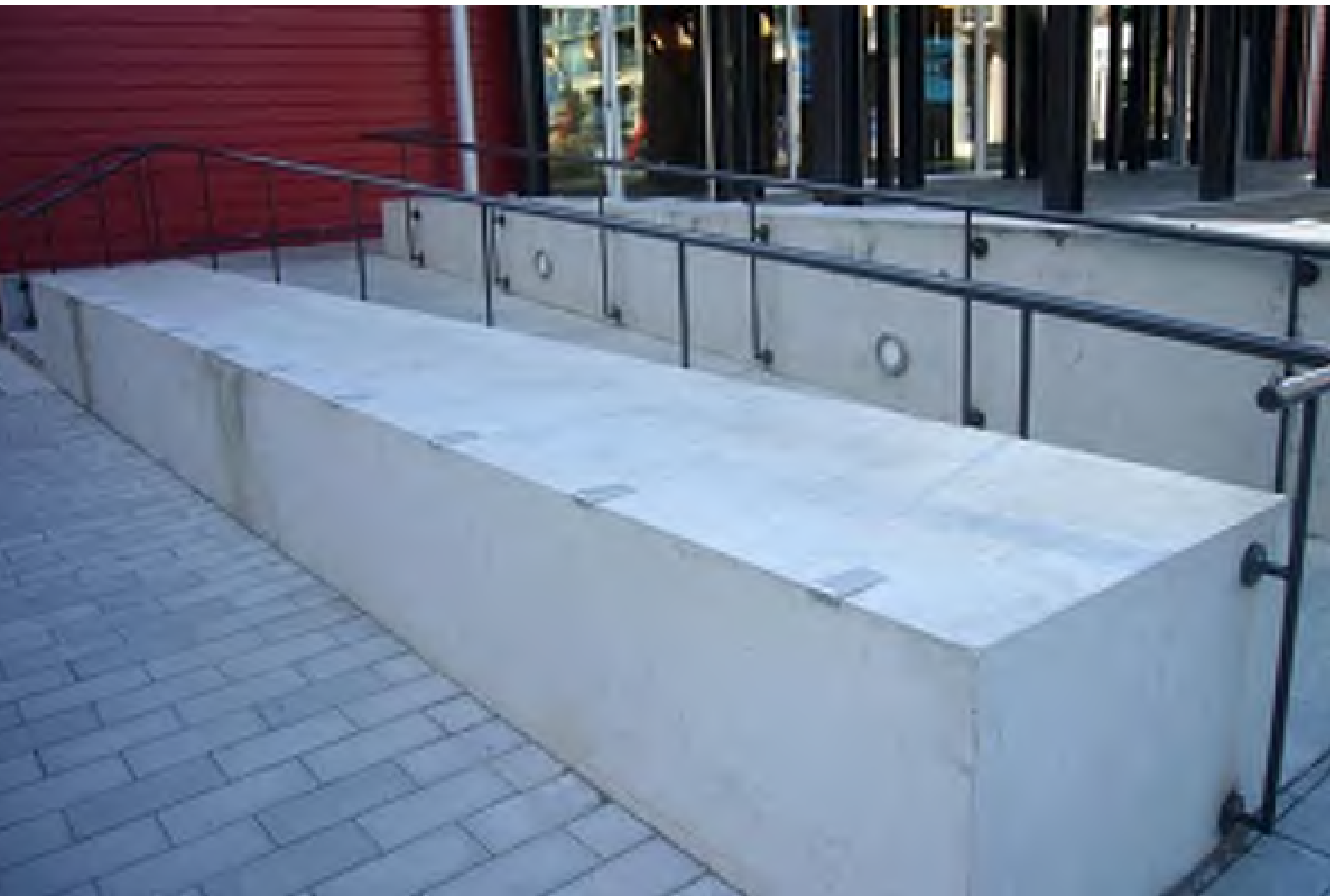
FLAT RADIUS SKATESTOPPERS EXAMPLE INSTALL
