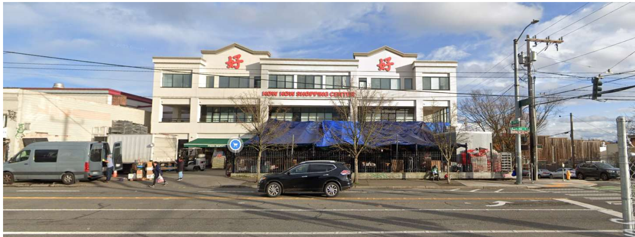
Existing West Facade Along 12 th Avenue S.
