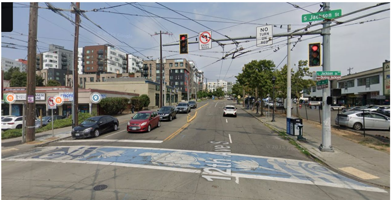
Existing condition of 12 th Ave S and S Jackson St north leg looking north
