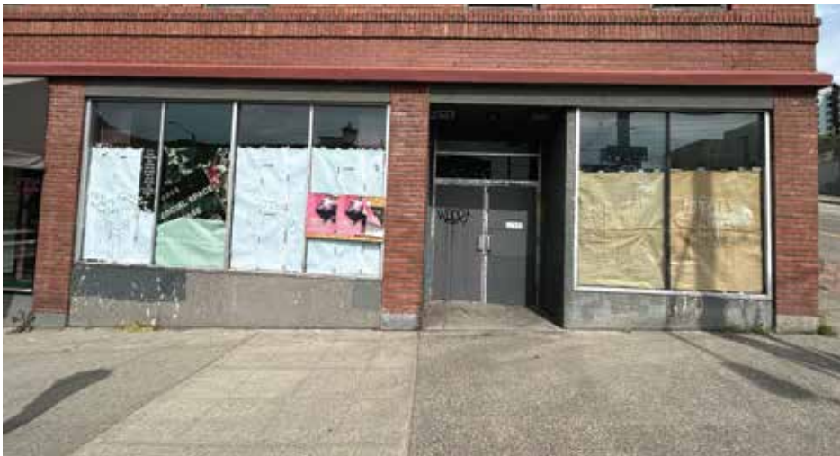
CURRENT CONDITION: Exterior
