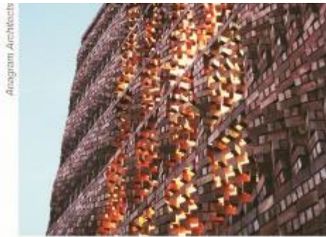
Bricks used for facade articulation
