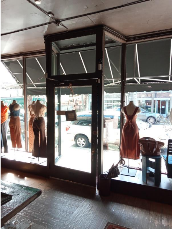
Inside view of the 5344 next door just to show the 1"x3" trim wrap on the door and transom window.
