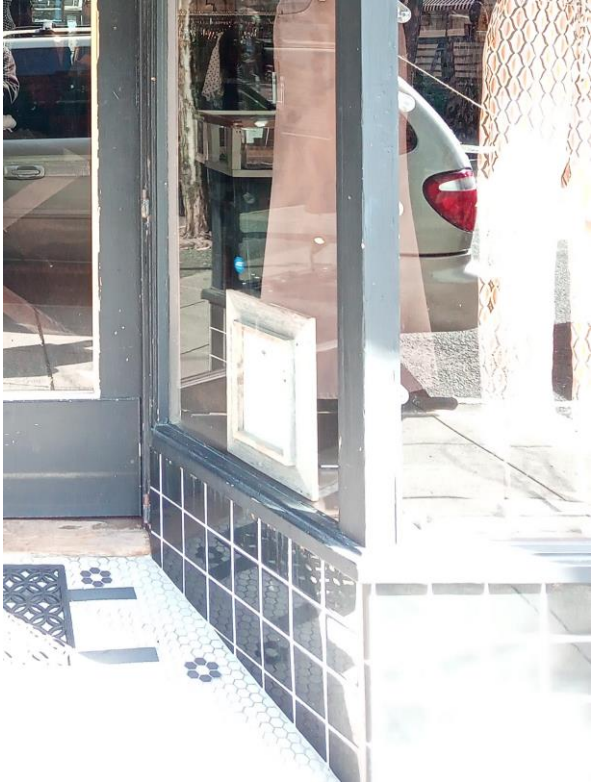
Inside view of the 5344 next door just to show the 1"x3" trim wrap on the door and transom window.
