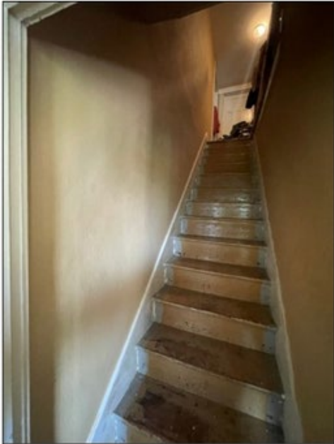
Missing Railing
