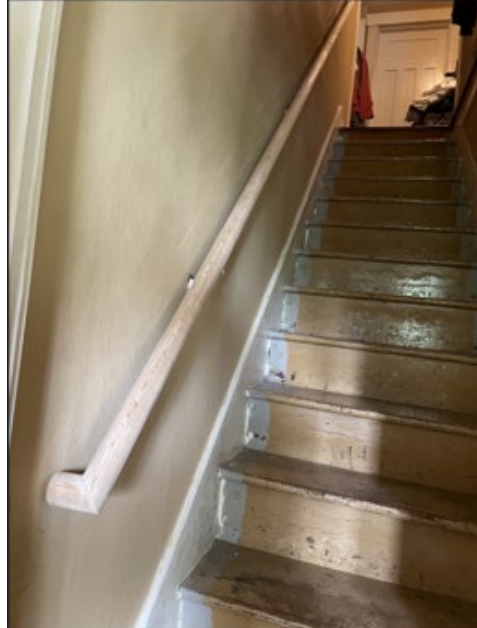
Installed Railing
