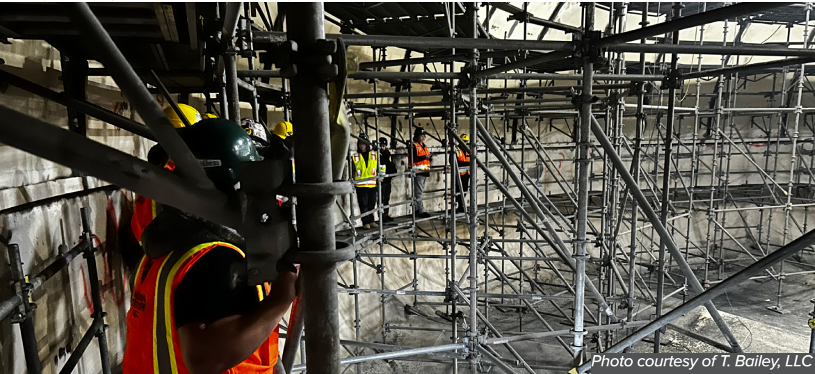
Photo: Students from the ANEW pre-apprenticeship program touring inside the Magnolia Elevated Water Tank project organized by T. Bailey, LLC, the general contractor on the project.
