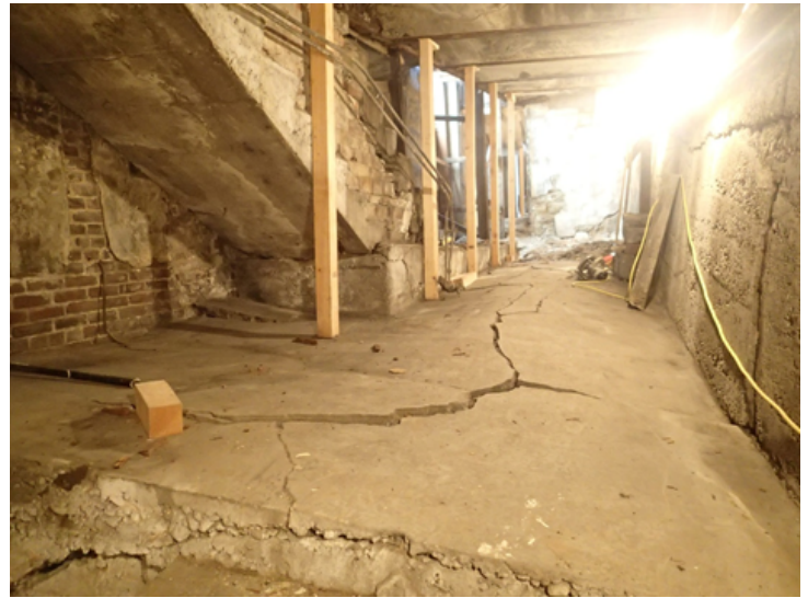
Columbia St Areaway with shoring being added
