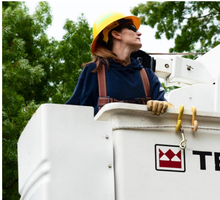
Crew conducting inspection/vegetation clearance around power lines.
