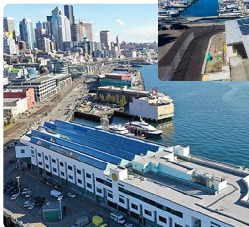
Pier 69 Solar Project
