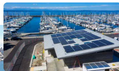
Shilshole Bay Marina Solar Project
