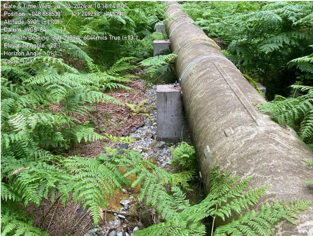
Looking north at ephemeral stream path on angular rock placed for erosion control on the west side of the penstock.
