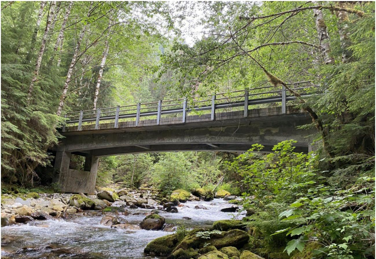
Figure 5. Concrete Bridge and Abutment over Newhalem Creek.
