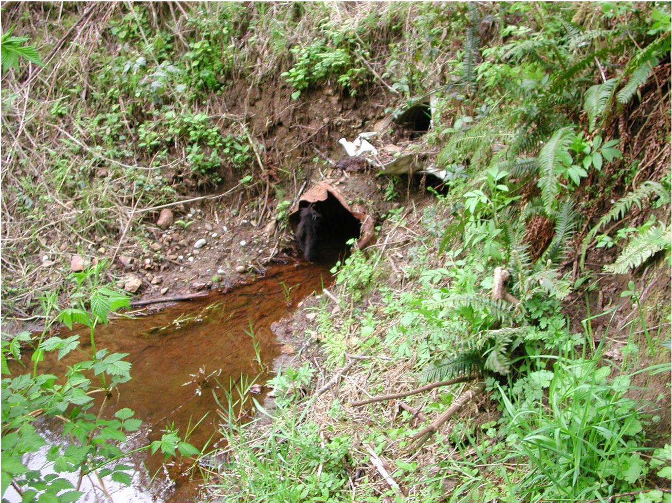
**Figure 3. Typical Stacked Culverts.**
