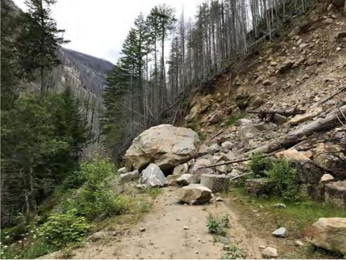
Figure 4. Rock slides along the dam access road. Older debris slide deposits are exposed in the right lateral scarp in the middle distance. (Source: City Light, 2022a).
