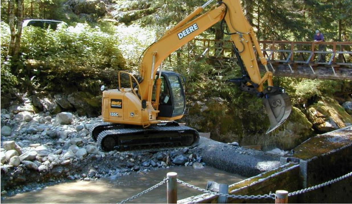
Figure 6. Annual excavation and downstream placement of accumulated sediment upstream of the diversion dam (year 2005) (Source: City Light, 2022d).
