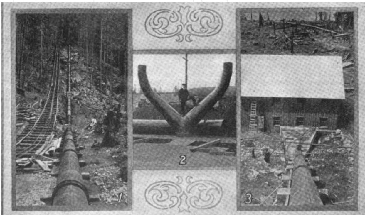
Figure 2. Views of electric arc welded pipe (*left*), Y-shaped pipe (*center*), and termination at powerhouse (*right*), 1921.
