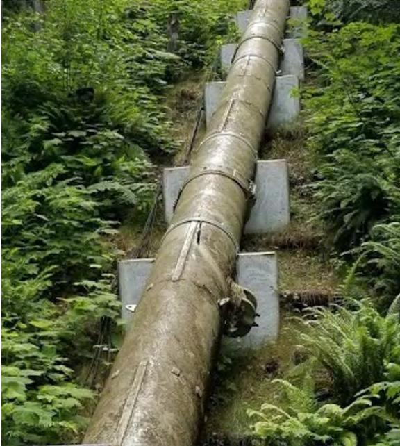
**Figure A-5. Penstock and Concrete Saddles**
