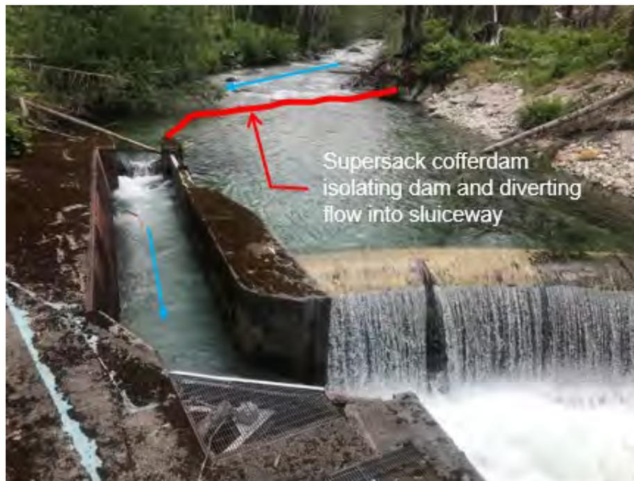
**Figure 2.2-4. Phase 1 dam removal approach – divert creek into right bank sluiceway.**
