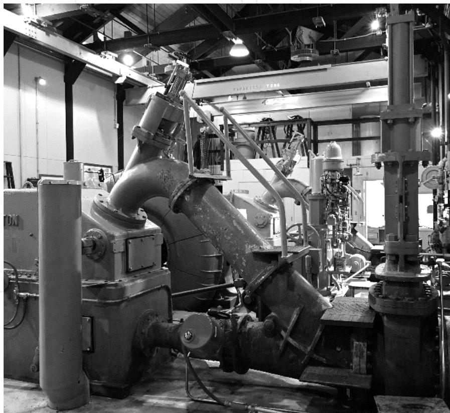
Figure 4. One side of double-hung Pelton unit showing new valves on double nozzle pipes, 2022.
