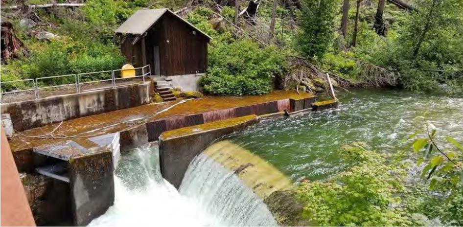
Figure A-2. Diversion Dam, Sluiceway/Intake, and Gatehouse
