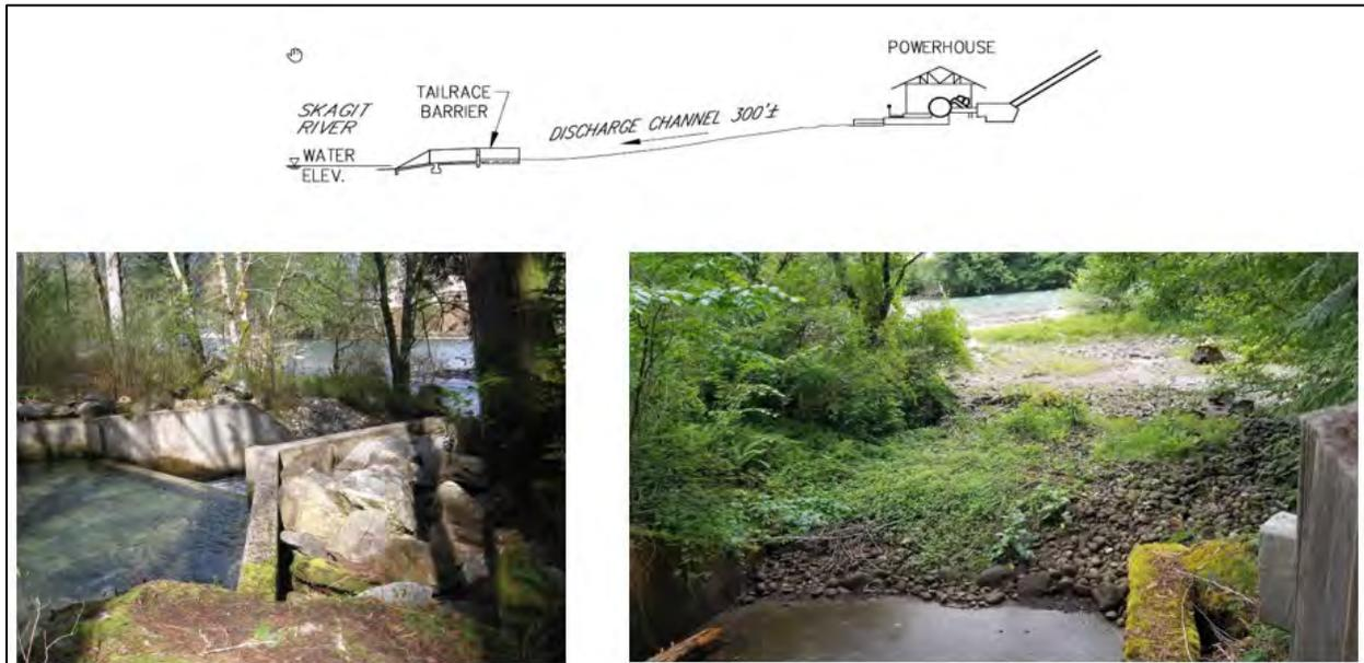
**Figure 2.2-10. Tailrace fish barrier (left), showing land separation from Skagit River (right; Skagit River in the distance).**
