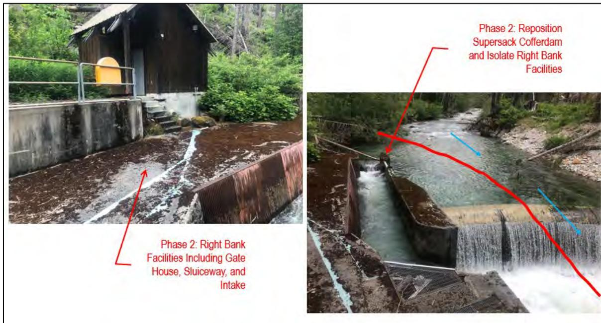
Figure 2.2-7. Right bank infrastructure to be removed during Phase 2.
