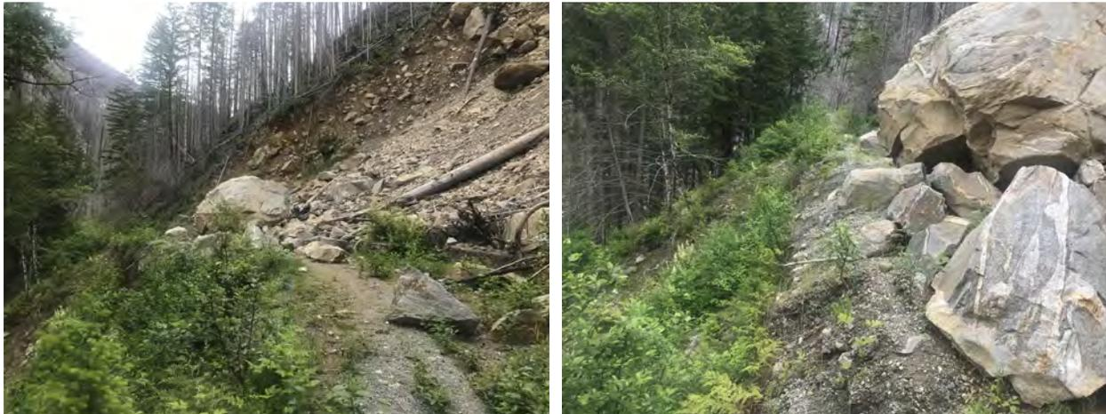
**Figure 2.2-1. Photos of Dam Access Road showing landslide and embankment instability.**
