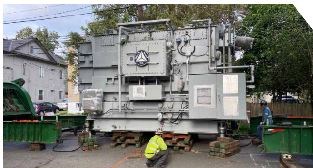
Transformer installment at East Pine substation
