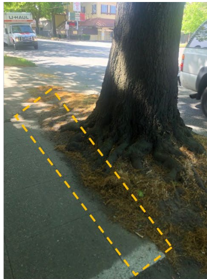
Street tree root structure encroaching on sidewalk near Lighthouse for the Blind.
