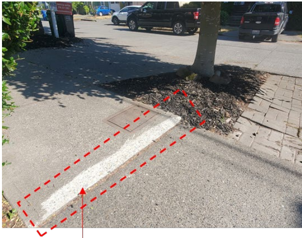
Example of a bevel : Edge of sidewalk was ground down so it matches the height of the neighboring concrete panel.
