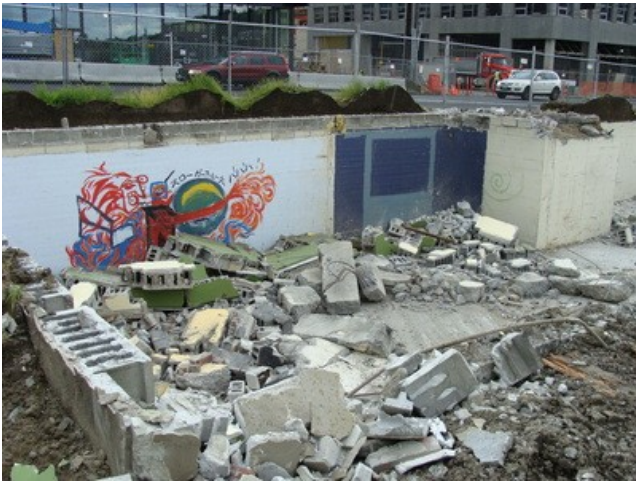
Mercer Corridor Project Building Demolition, April 5, 2010 Item 168662, Seattle Municipal Archives
