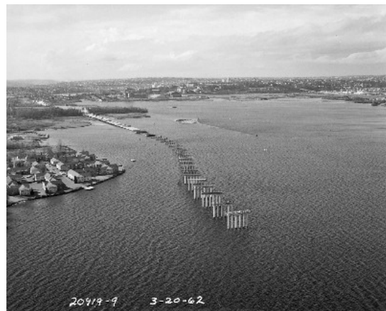
Construction begins on the SR 520 bridge over Lake Washington. March 20, 1962
