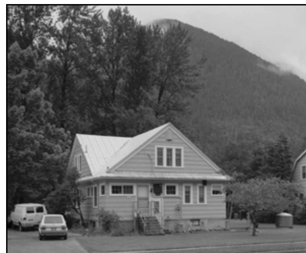
North facade, house no. 7, Silk Stocking Row, Newhalem, 1990. Skagit Power Development, Skagit River & Newhalem Creek Hydroelectric Project. Library of Congress, Photos from Survey HAER WA-24.
