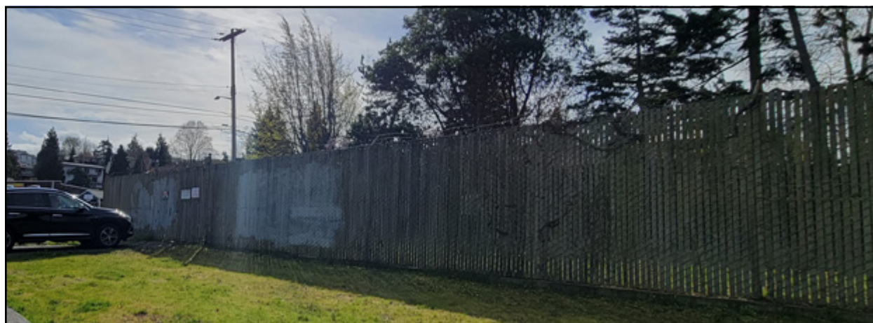
Former Dumar Substation— 1605 SW Holden St. (photo: Kate Clark).
