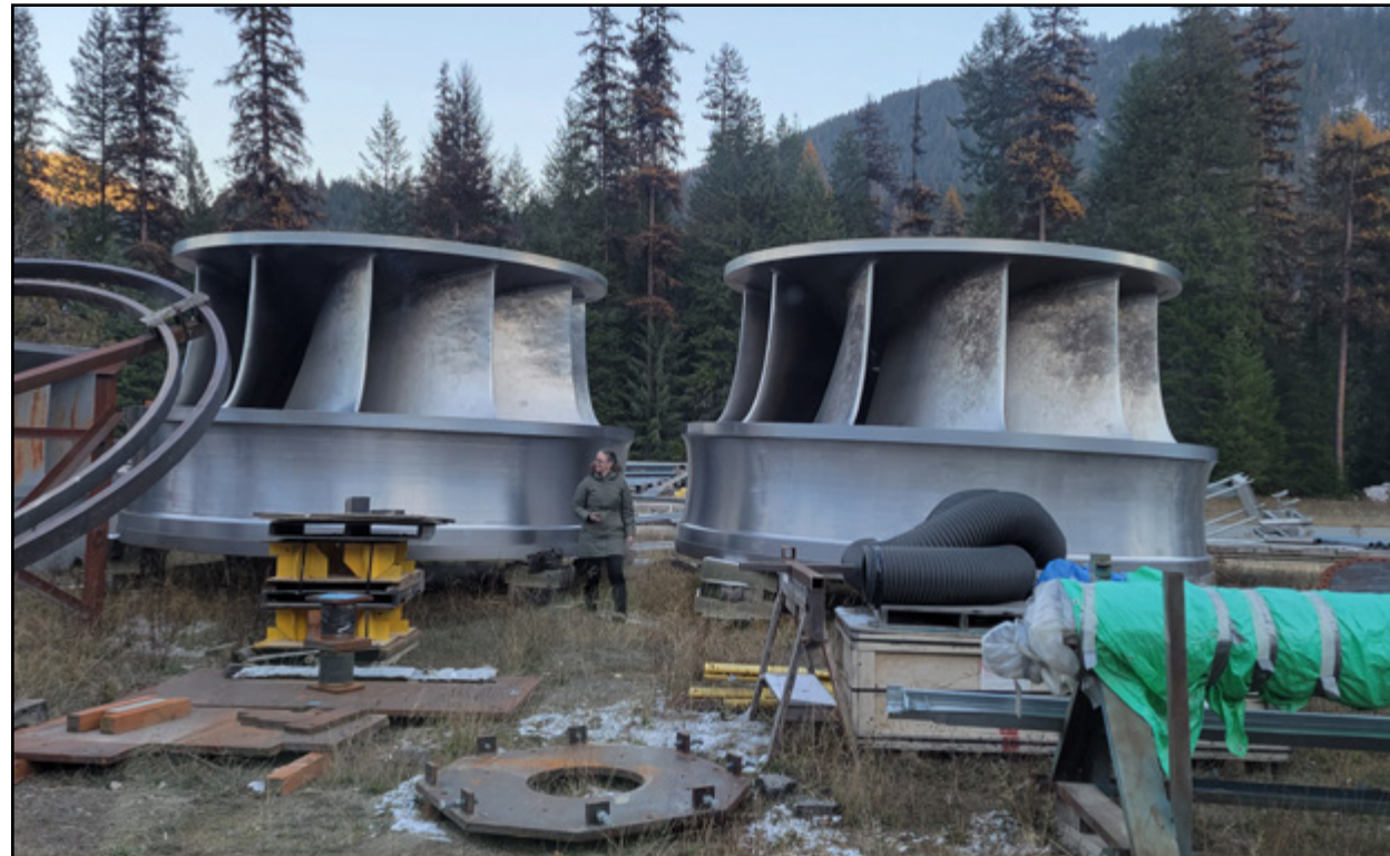
Seattle City Light salvage turbines, Boundary Facility (photo: Kate Clark).
