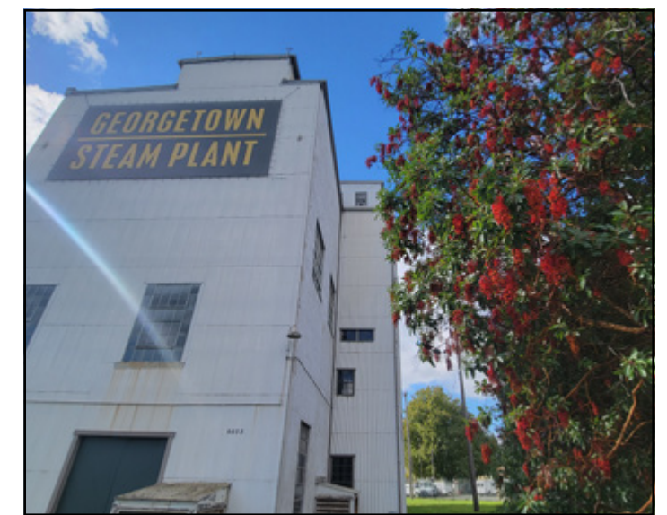
Georgetown Steam Plant (photos: Kate Clark).
