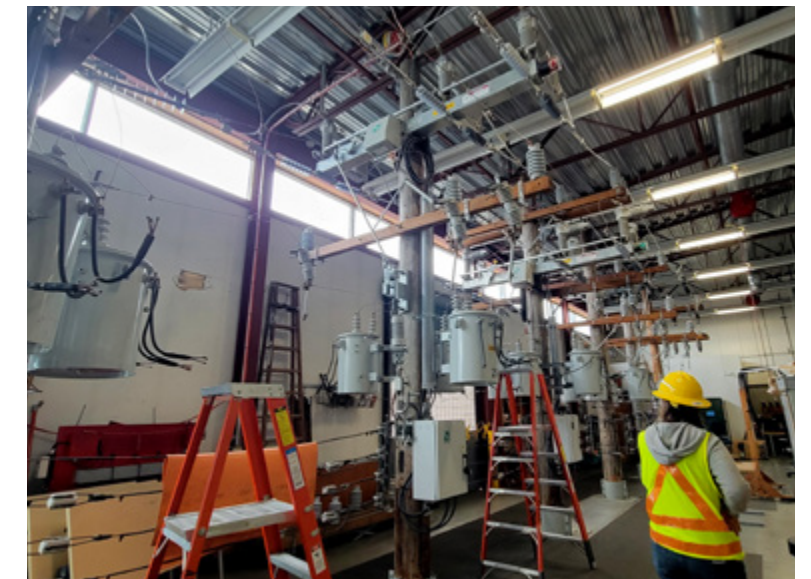
Tour of Seattle City Light Apprenticeship facilities at the South Service Center.
