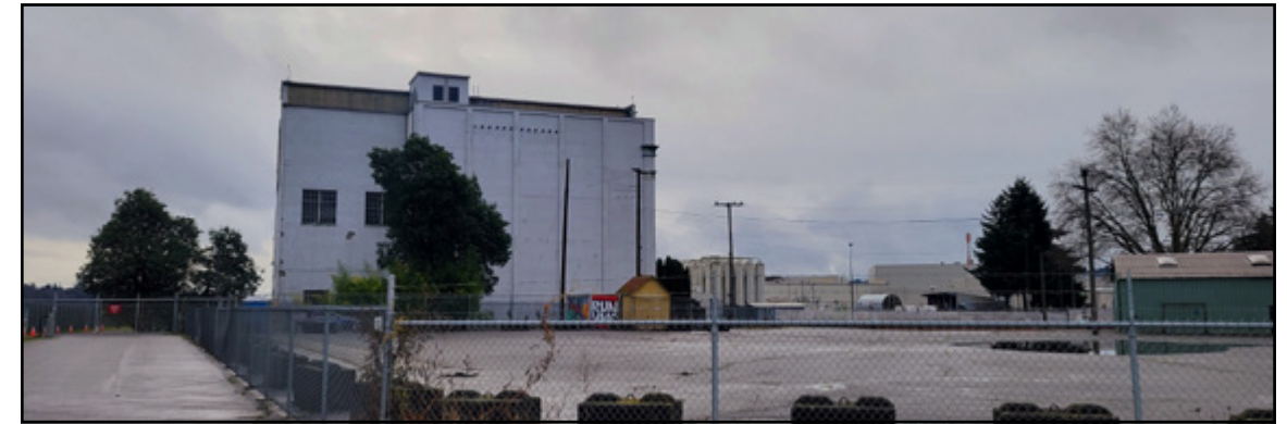
Georgetown Steam Plant Temporary Fence Entry. Photo: Kate Clark.
