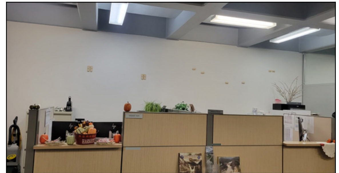
Office wall, Boundary Facility, 2022 (photo: Kate Clark).
