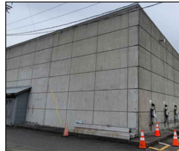
Building N, Seattle City Light South Service Center (photo: Kate Clark).
