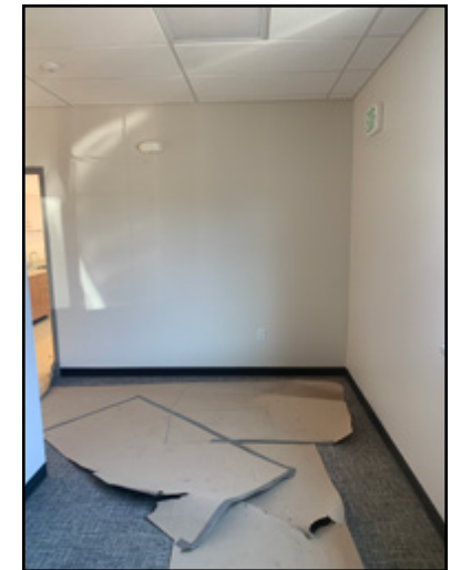
Interior view of Admin Building entry wall.
