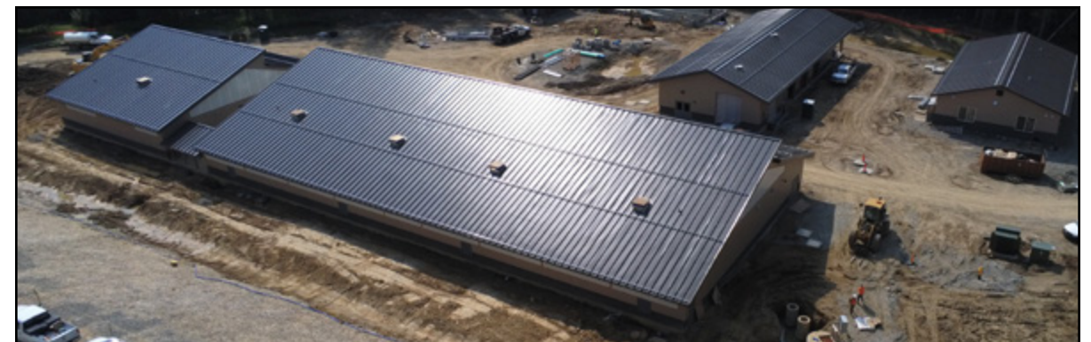
Aerial view of Usk Hatchery Admin Building mid-construction.
