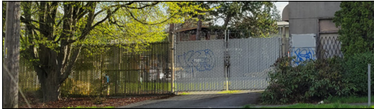
Former Roxbury Station— 9460 34th Ave SW (photo: Kate Clark).
