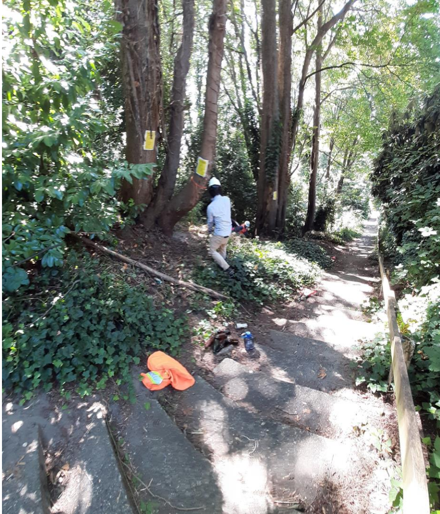
Pre-Restoration Treatment – August 2020
