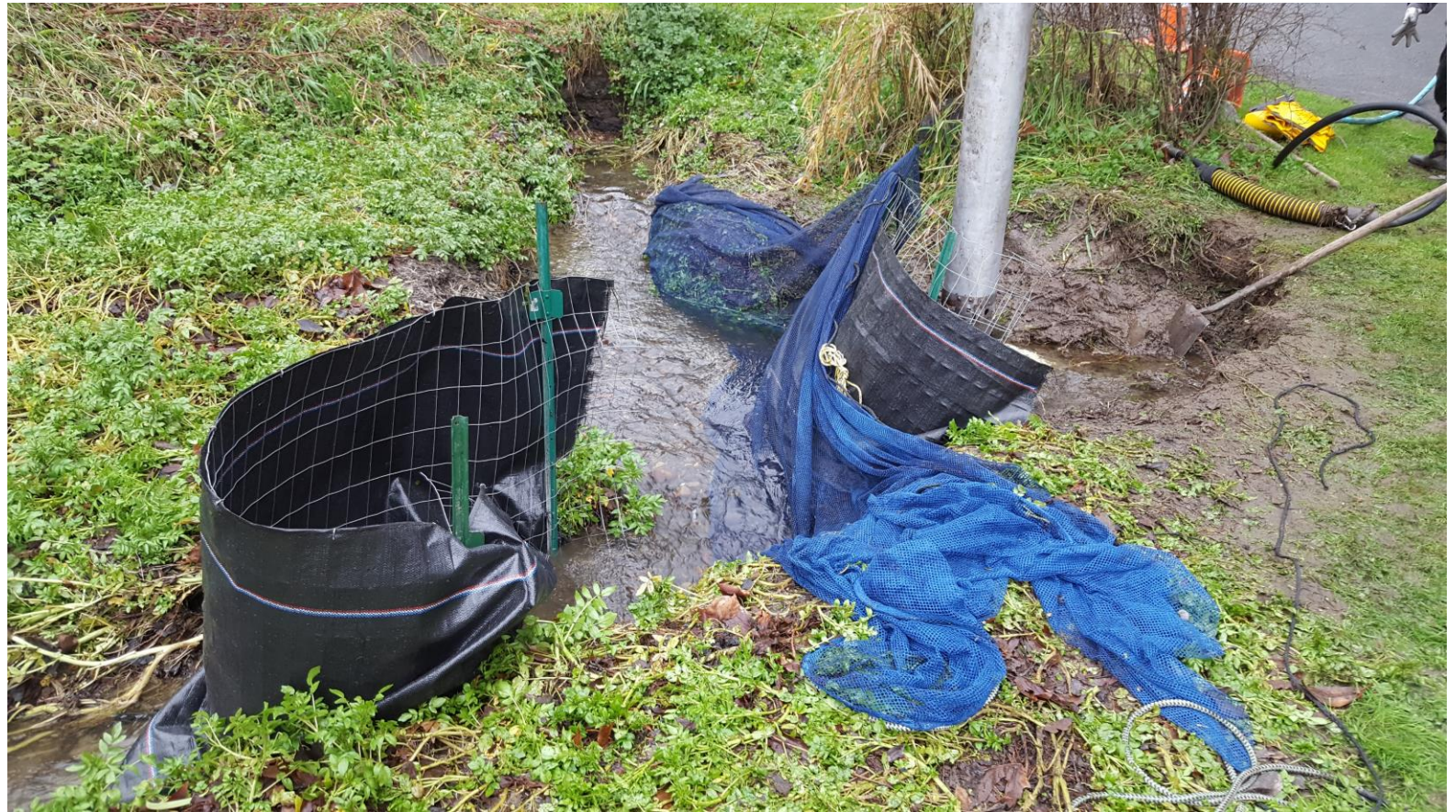
Emergency SPU Operations – Dredging and Bypass in Lower Maple Creek– December 2019
