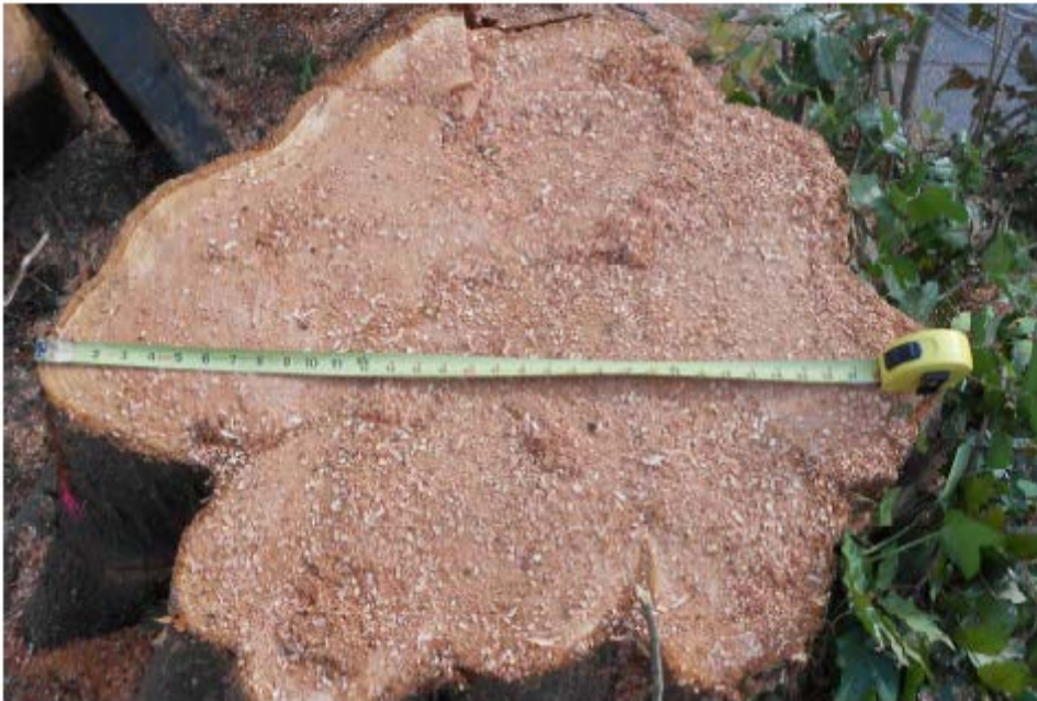
Remaining stump after Western Red Cedar was removed November 25, 2012 without notifying DPD. Note diameter is at least 35 inches.
