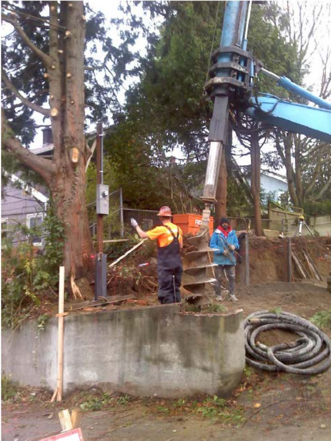
Workers allegedly “saving” the Western Red Cedar at 5201 Phinney Avenue, November 14, 2012. Note the deep excavation within the root zones of all the three trees to be preserved along the western property boundary.
