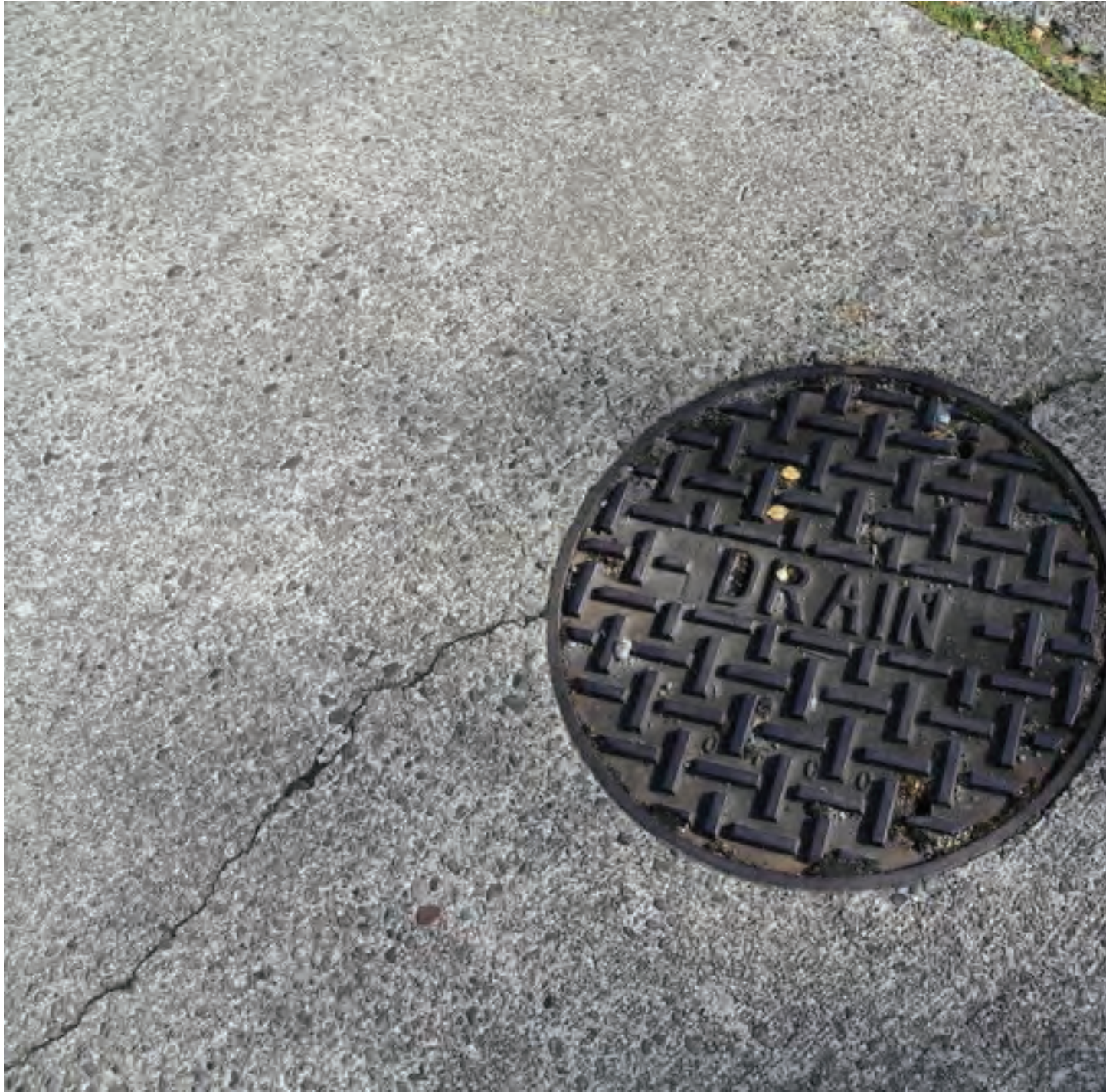
Storm Drain – separated from sanitary sewer mainline.
