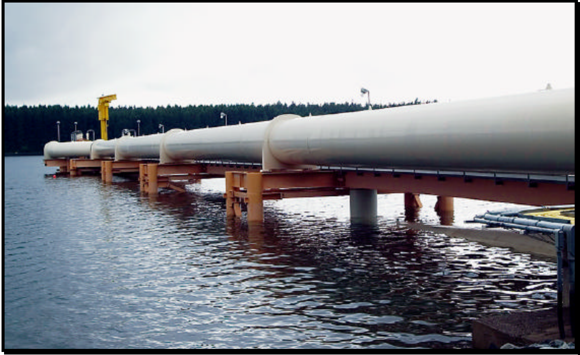
Intake Structure in Lake Youngs
