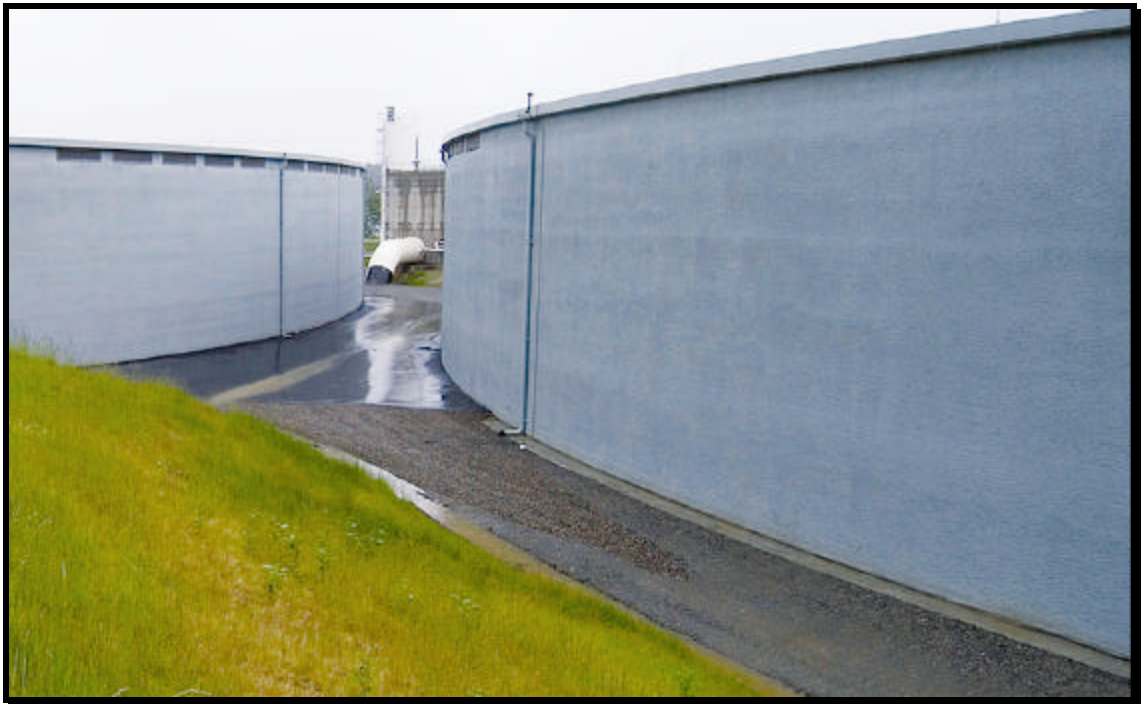
Treated Water Tanks
