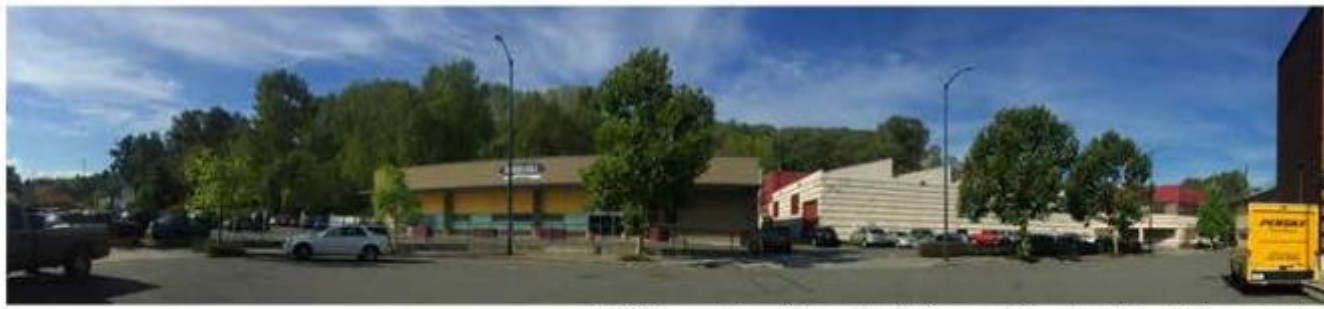
UW laundry, King Hall & parking behind the station
