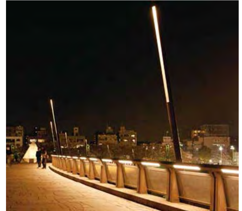
Bridge mounted lighting
