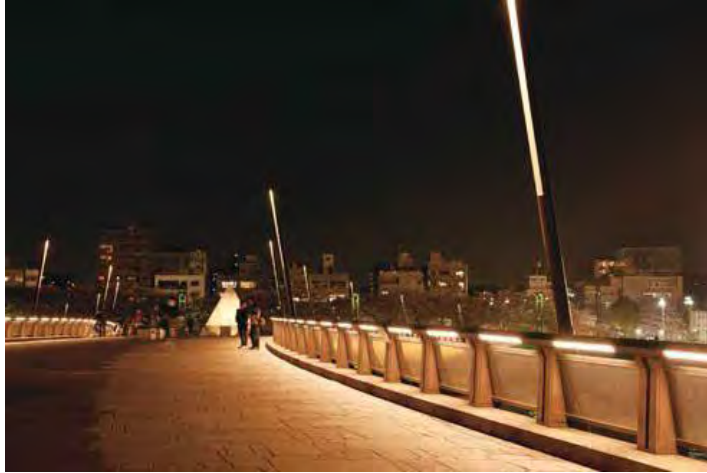
Higher overpass railings with integrated lighting
