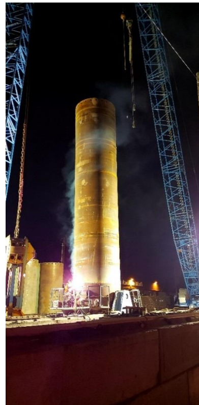
Crews weld shaft casing for Lander Bridge
