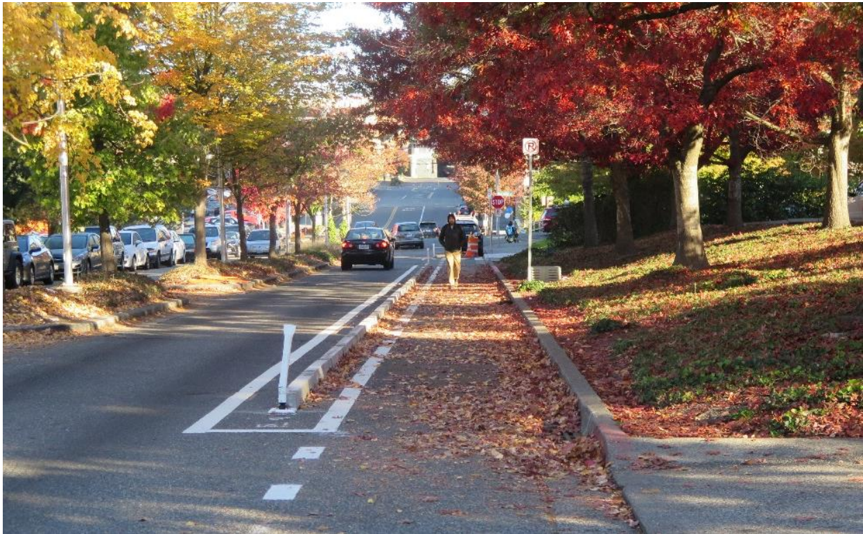
Low-cost sidewalk on 3rd Ave NE
