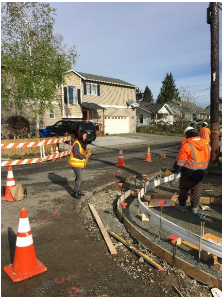
Forming new curb ramps and sidewalk corner
