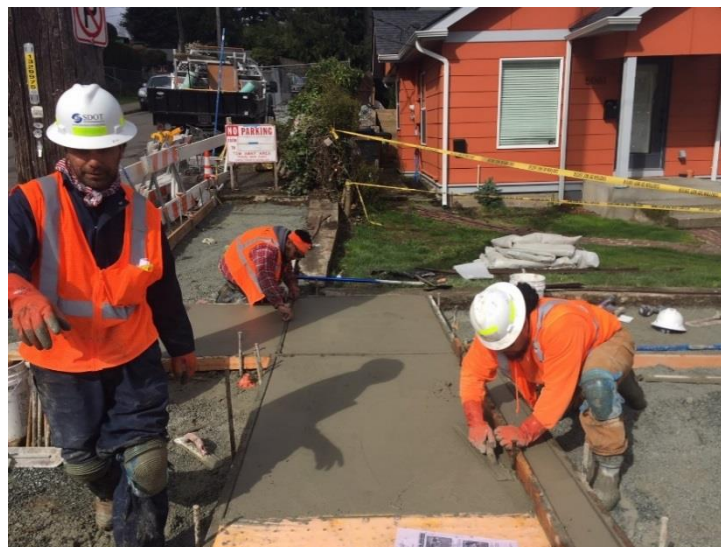
Crews building sidewalk
