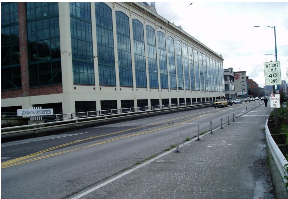
Existing conditions on Fairview Ave N
