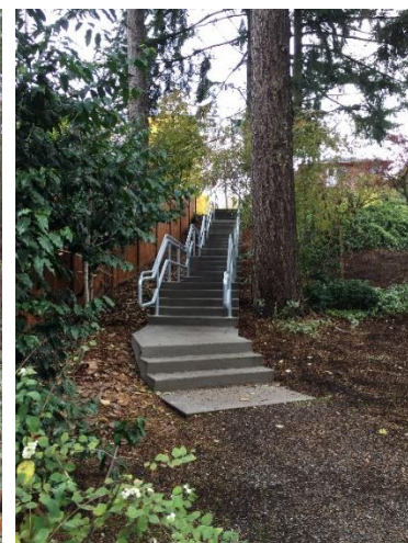
N 88th St stairway, after
