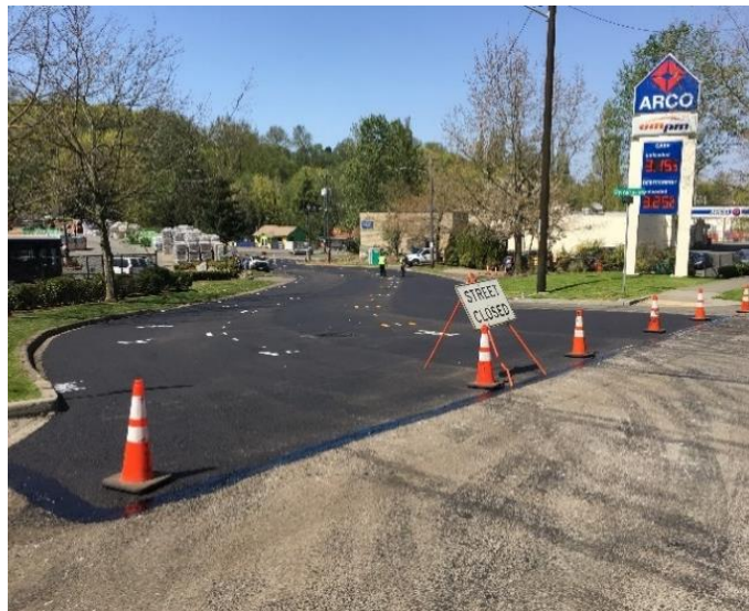
Pavement after repair
