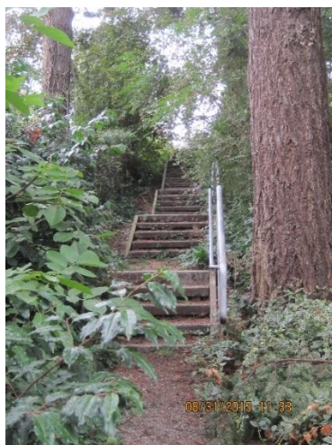
N 88th St stairway, before
