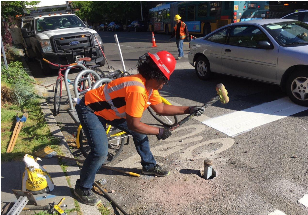
Crew intalls bike parking
