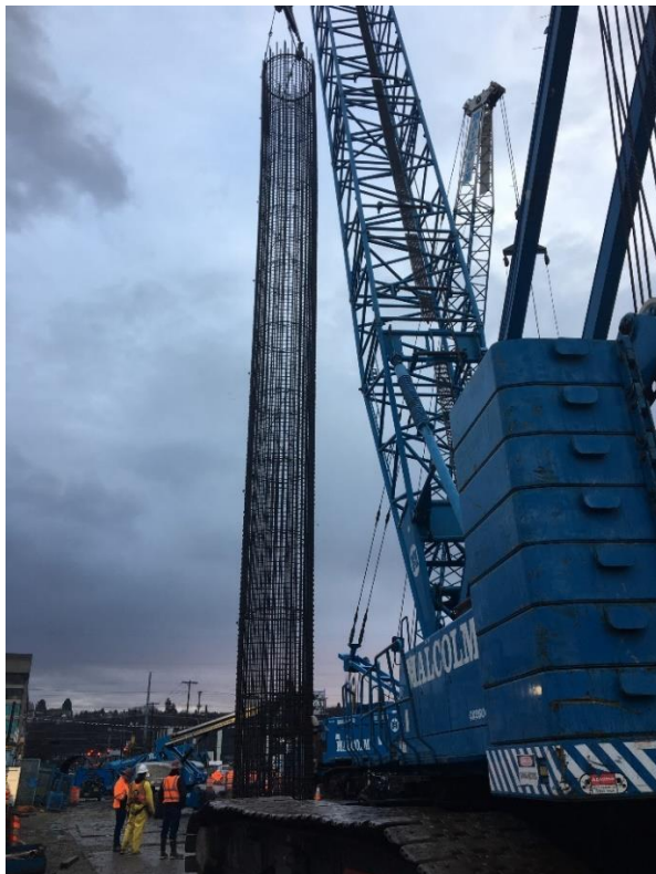
Crane sets rebar cage for Lander Bridge shaft casing
