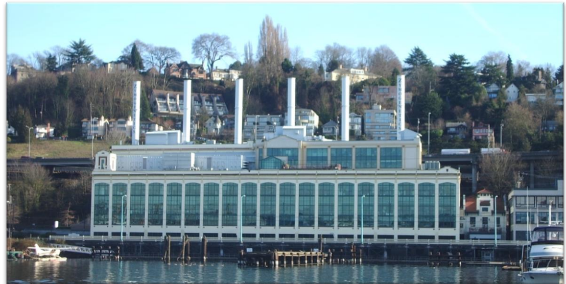
Fairview Ave N bridge is next to historic Union Steam Plant building (ZymoGenetics)
