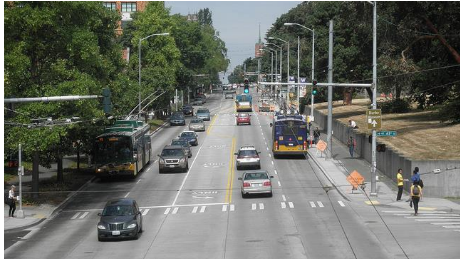
15 th Ave NE paving project (completed)
