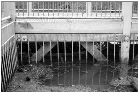
Overflow riser – close-up of drop intake with pond overflow into bypass.
