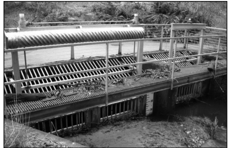
High-flow diversion structure.
