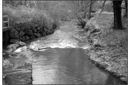
Thornton Creek main stem at high-flow diversion structure. Residents should take extra precautions to guard against flooding, if their home is near a creek.
