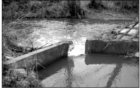
Meadowbrook Pond outlet and flow control weir (Outlet Weir B), with the main stem of Thornton creek in the background.
