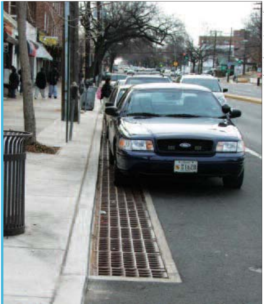
A gutter filter cleanses runoff before sending water to the stormdrain.
