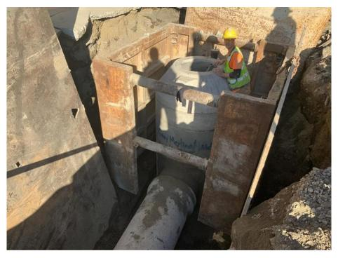
Figure 4-6. Central Waterfront Construction – Maintenance Hole Installation
