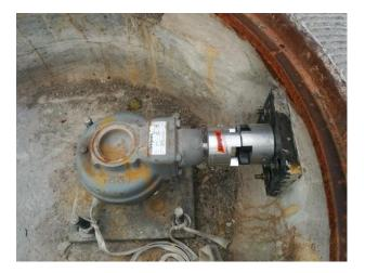
Figure 4-1. New Basin 99 Sluice Gate (left) and Actuator Motor (right)
