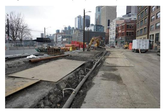
Figure 4-5. Central Waterfront Construction – Dewatering System
