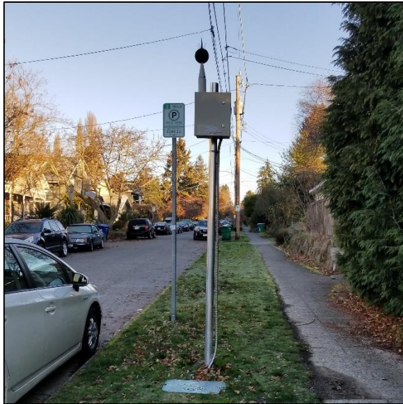
Photo 1. Equipment at Location 1
