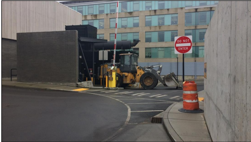
Photo 3. Loader at Fueling Station
