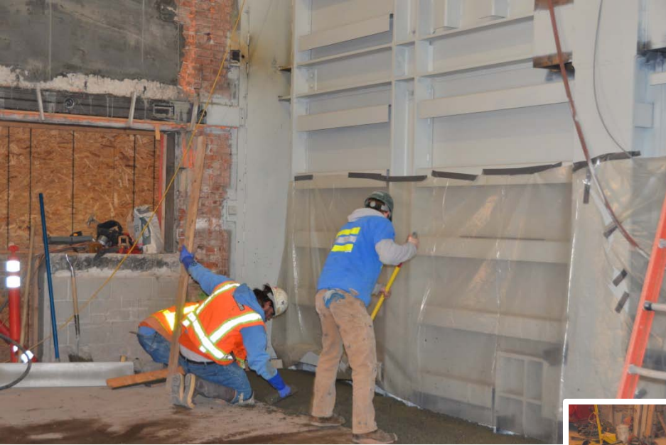
Grade beam for the shear wall outside the original Women's Waiting room was casted on site.
