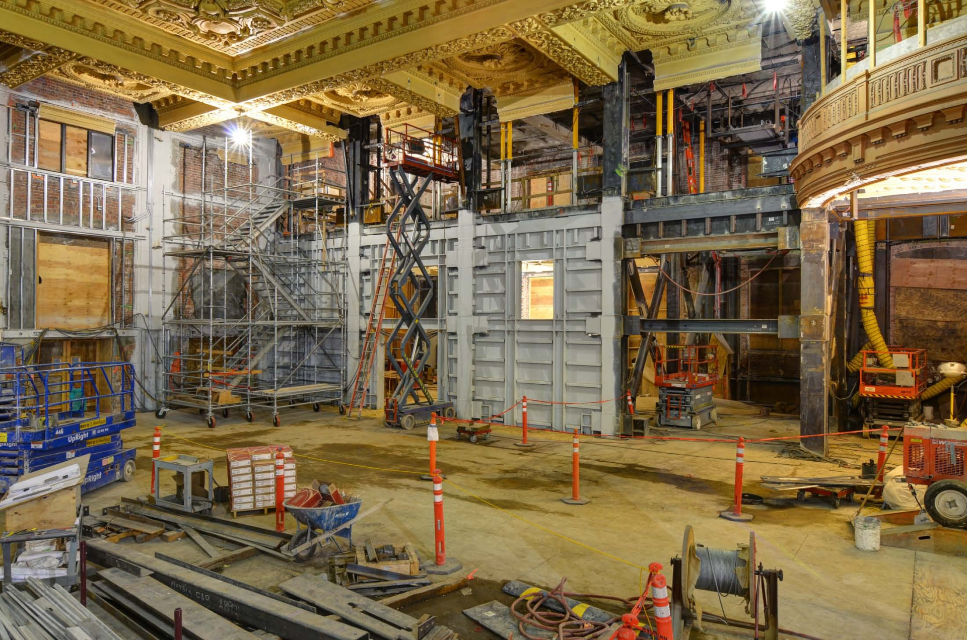
New steel columns, beams, trusses, bracing, piles and decking ensures the structural steel of the station are connected to withstand future seismic forces.
