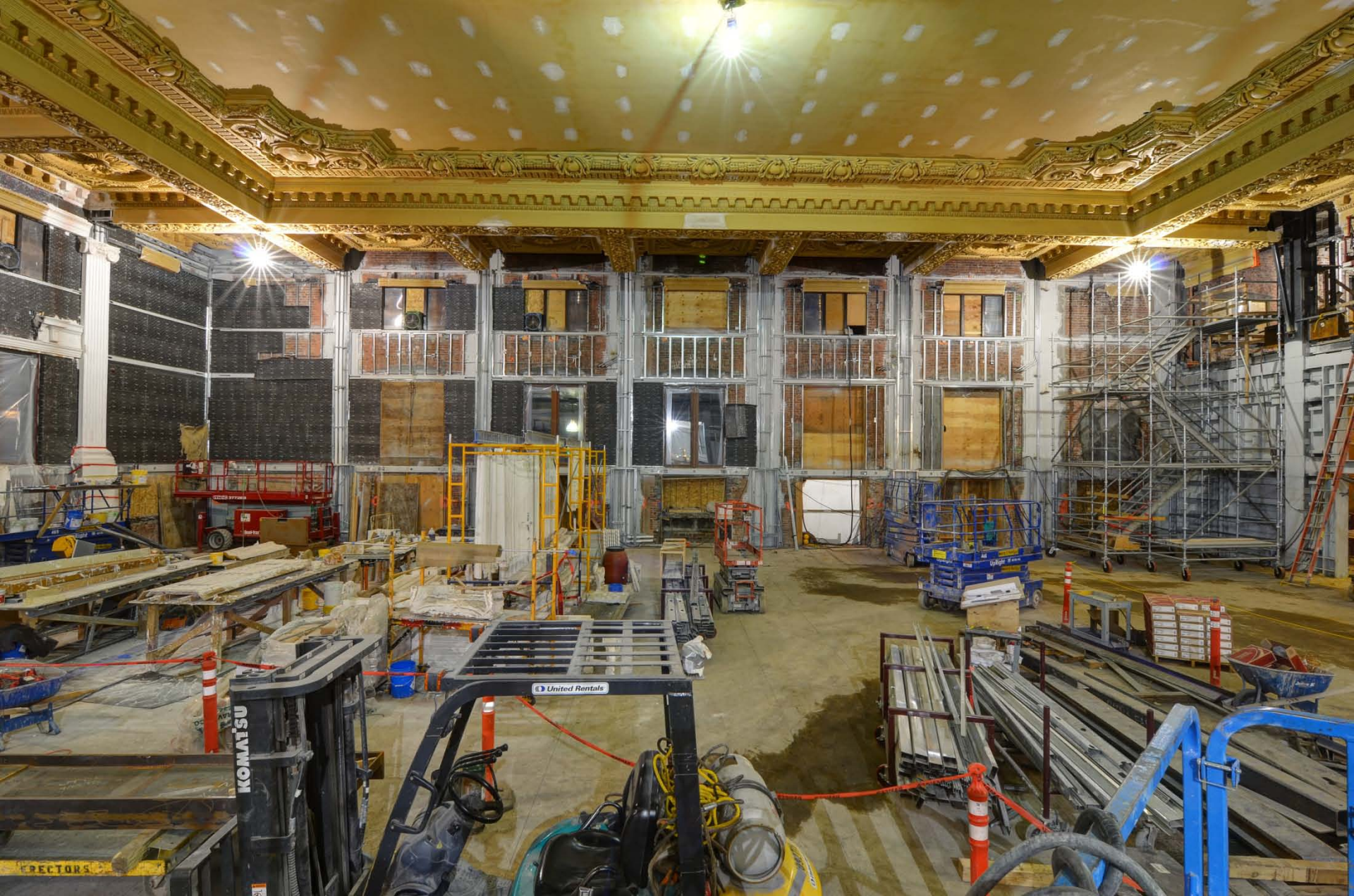
A wide angle view towards the south wall of the station terminal. Metal lath is going up on top of the black wall area in preparation for plaster installation.
