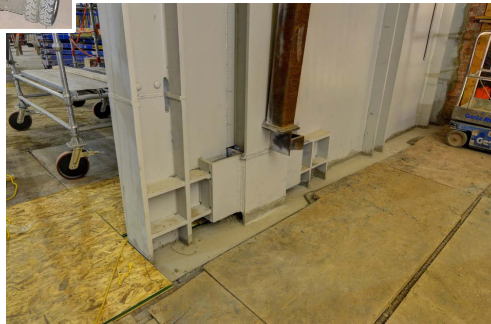
Both the grade beam and shear wall are tied to the reinforced concrete piles for stability/anchorage.
