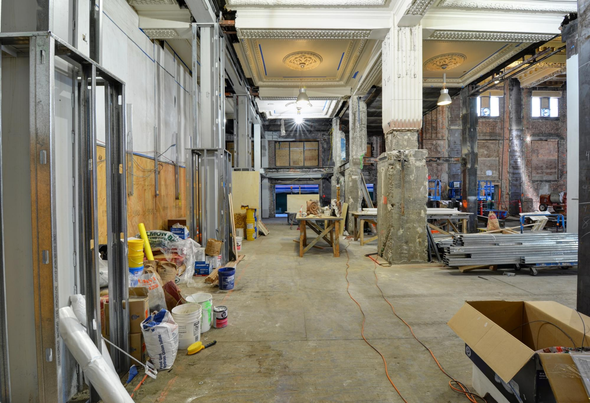
Temporary wall on the left separates Amtrak current operating space from construction zone.
