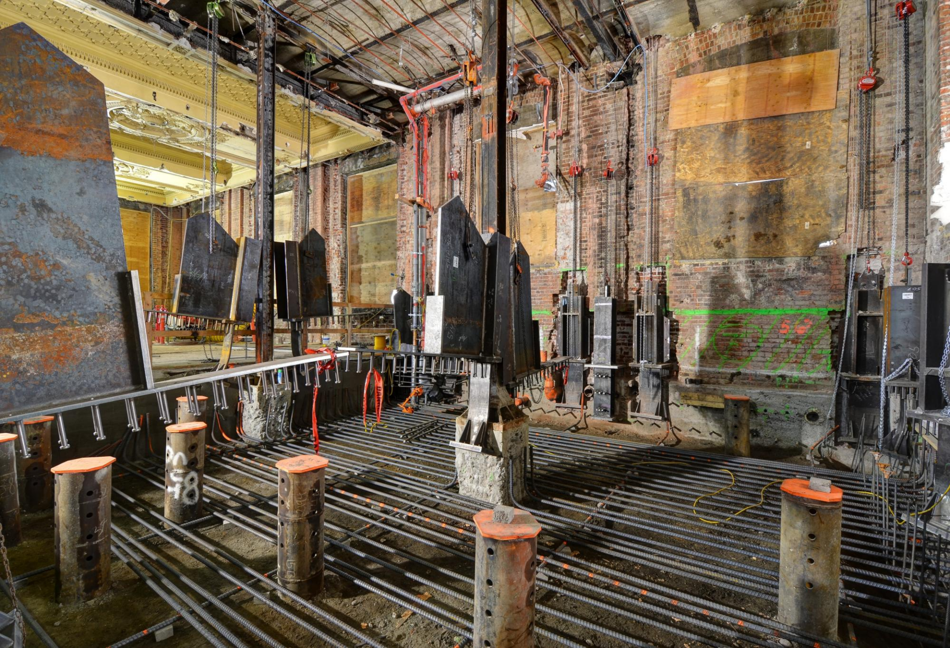
This area will have new deep pile foundation, columns, grade beam, along with new plumbing.
