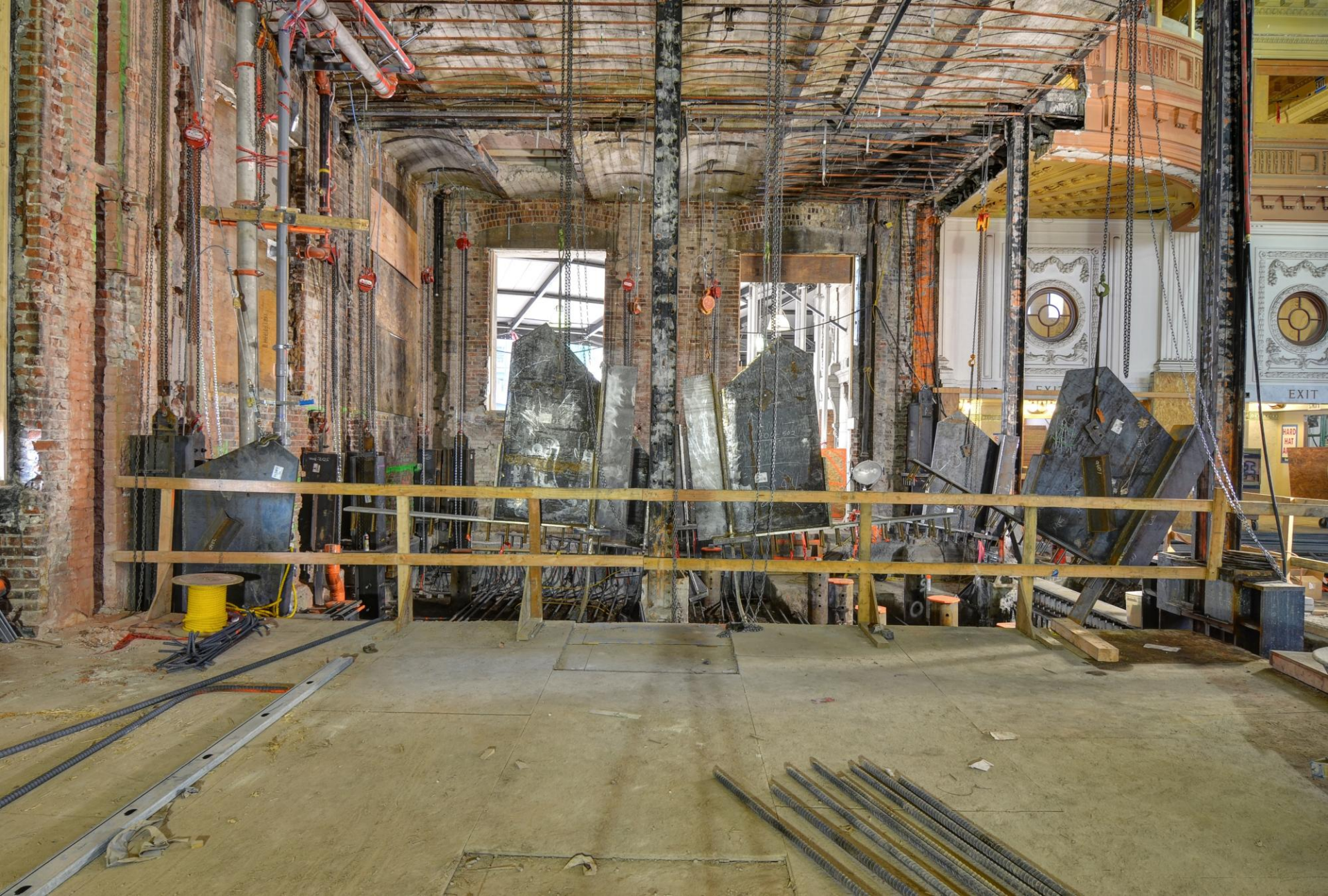
A collection of new steel pieces which will be installed as part of the seismic upgrade.
