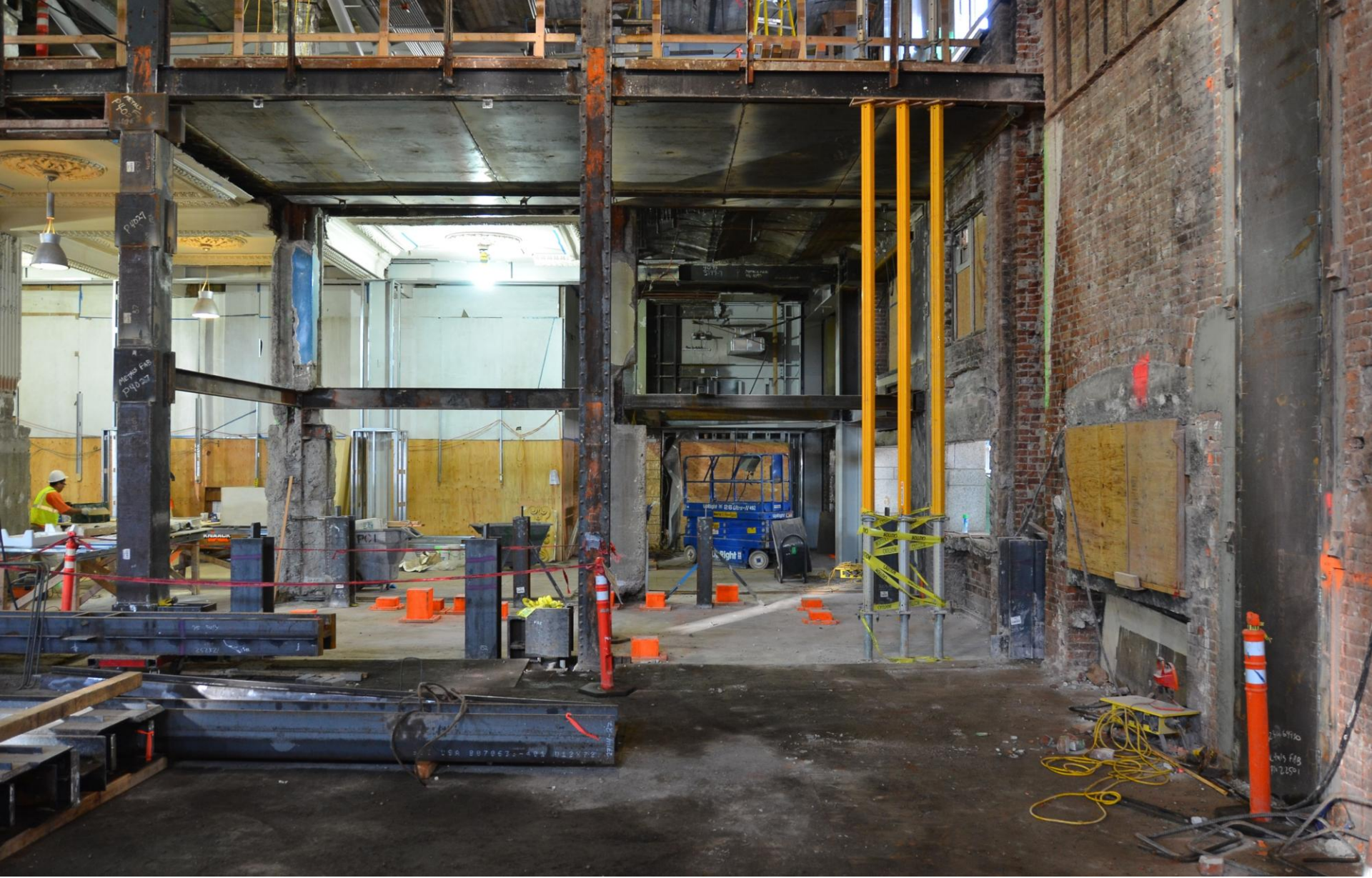
New steel framing at previous Amtrak lunch room provide additional structural load capacity. New concrete slabs, deep pile foundation, grade beam, and new utility lines were also installed.
