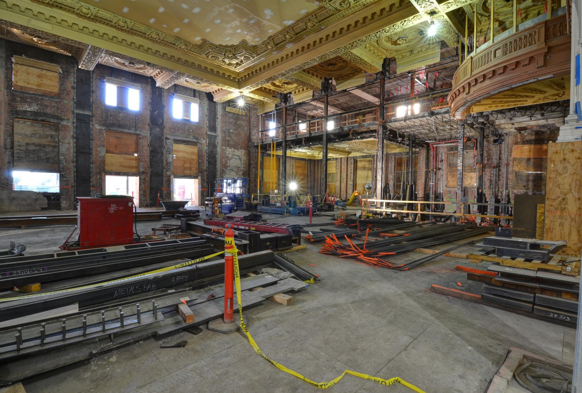
Looking northwest from the main waiting room. Top left: Large sheets of metal enclosed newly installed columns to support the building's vertical and shear stress.
