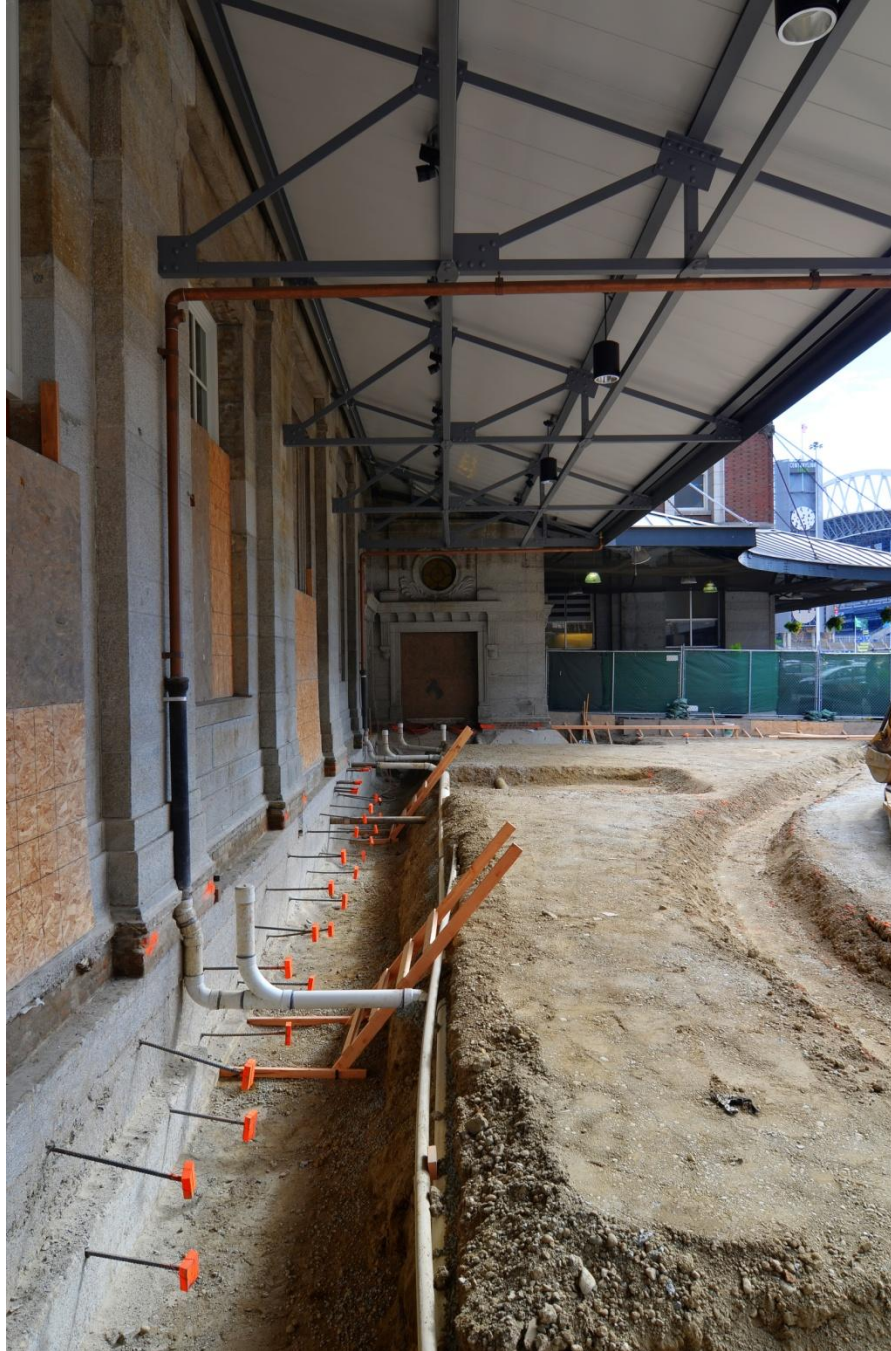
Excavation on the station's west side for foundation improvements.
