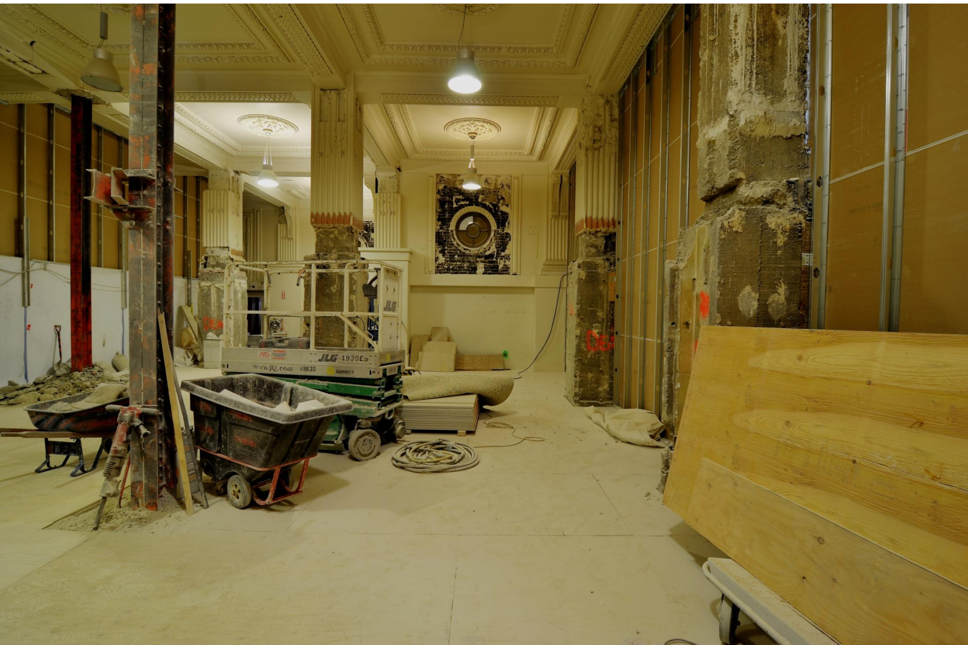
Concrete was removed from the supporting columns to prepare for installation of additional structural steel.
