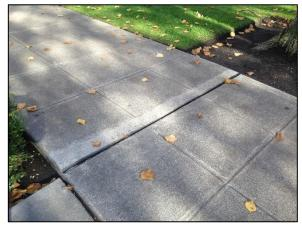
Beveling (or grinding) Sidewalk Uplift to Make Smooth Sidewalk Transition
