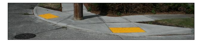
Curb ramps are an integral part of an accessible pedestrian network. They ensure sidewalks and street crossings are usable to people who use wheelchairs or have other disabilities. Because sidewalks are typically located higher than the roadway, a ramp or sloped surface is needed to connect pedestrians to the crosswalk.
