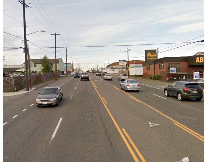
Looking north on Aurora Ave N (SR 99), near the intersection of N 92nd St
