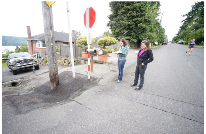
Existing conditions at the southeast corner of the intersection of 37th Ave NE and NE 145th St
