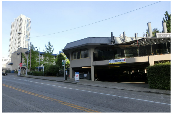
Existing conditions at the Intersection of Erickson Pl NE and 35th Ave NE
