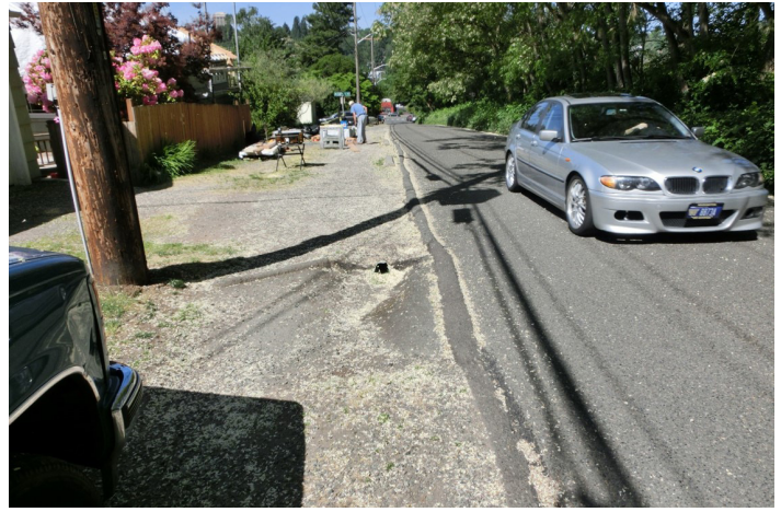
Utility poles may need to be relocated to the planting strip to avoid creating a barrier in the proposed sidewalk.
