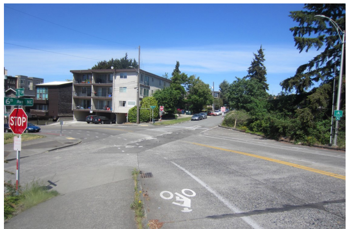
Existing Conditions at NE 70th St and 6th Ave NE.
