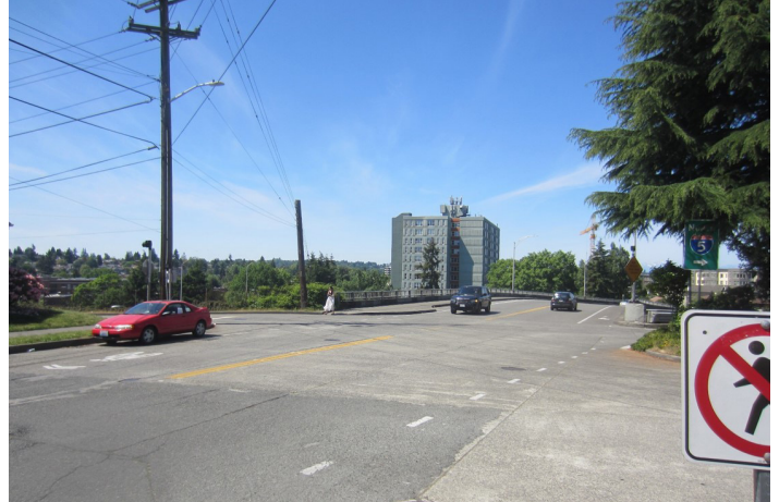
Existing conditions at NE 70th St and 8th Ave NE.
