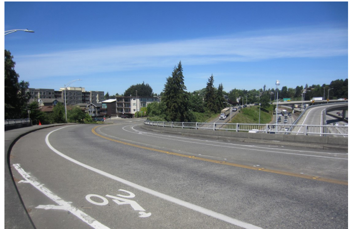
Existing conditions on overpass section of NE 70th St.
