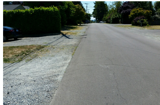
Looking south from the east side of 39th Ave SW north of SW 102nd St
