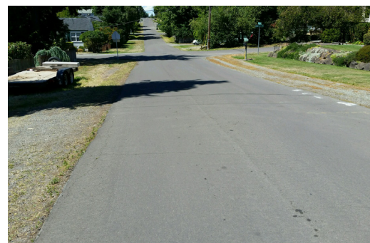
Looking west from the south side of SW 104th St east of 40th Ave SW
