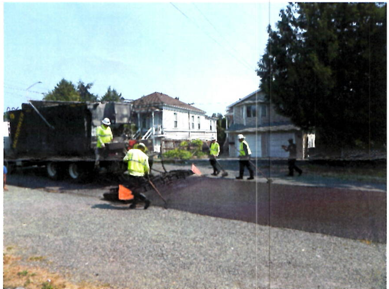
Example of the slurry seal process
