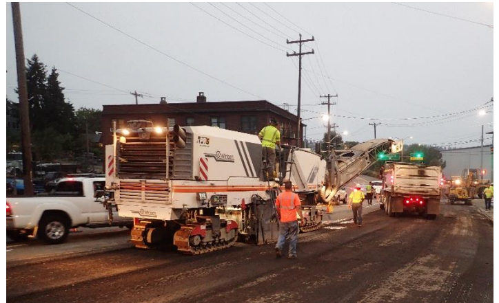
Example of crews grinding the street
