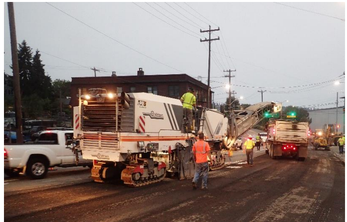
Example of crews grinding the street
