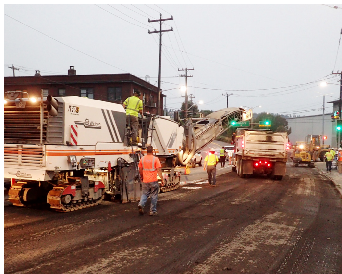
An example of crews grinding
