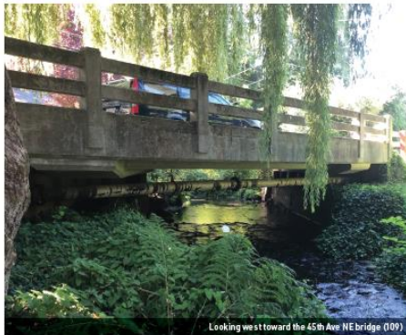
Looking west toward the 45th Ave NE Bridge (109)
