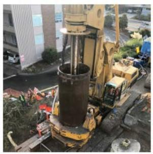
LEFT: An oscillator will be used for drilling shafts. This method causes minimal vibration.
