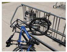
Rack does not provide 2 points of support or place to lock to frame (Photo: MIGISvR)
